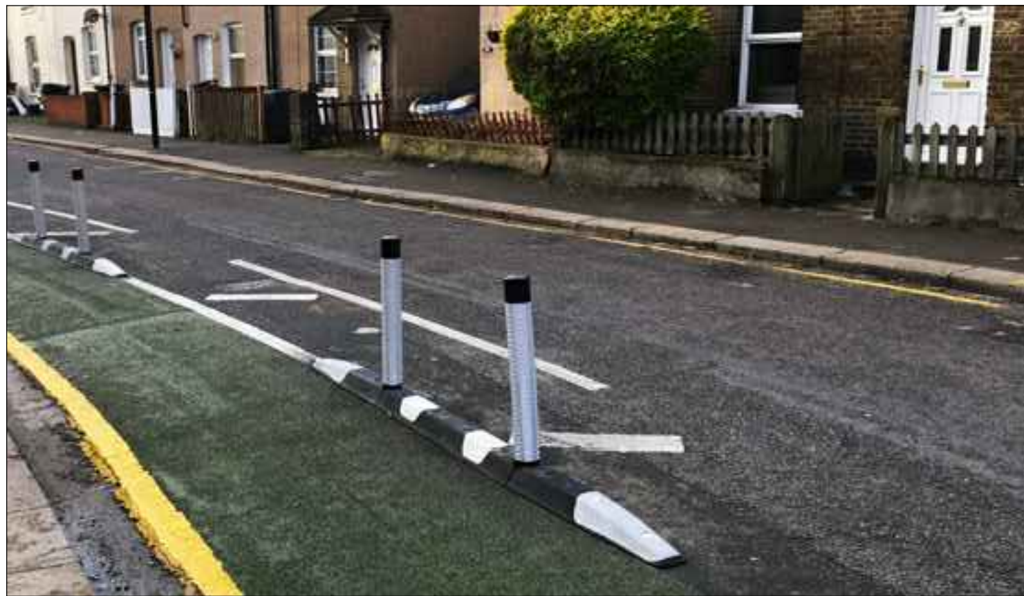
GREENWICH ORCA WANDS - 2.5m LONG SEE DRAWING COM-12727-1100-01 FOR CONSTRUCTION DETAILS http://www.rediweldtraffic.co.uk/products/cycle-lane-products/greenwich-wand-orca/
