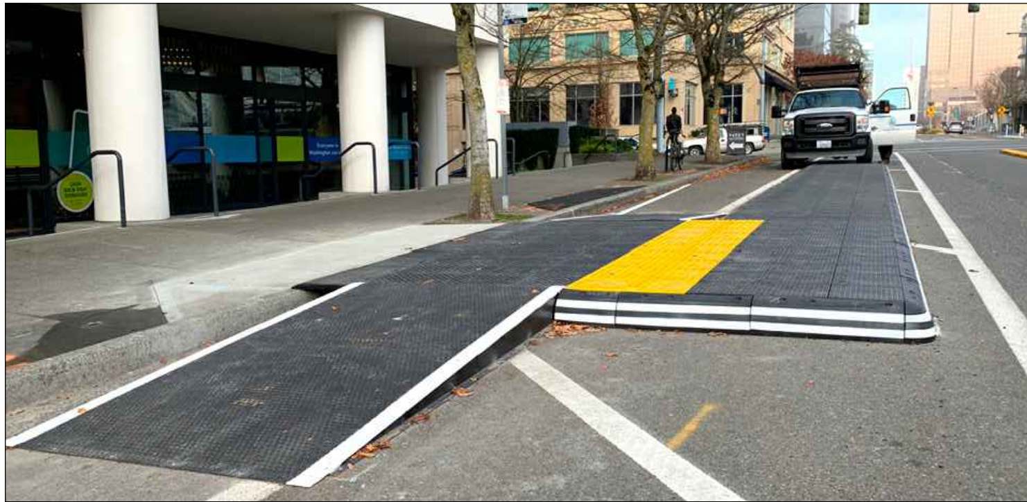
VECTORIAL FLOATING BUS STOP - ONE TO BE LOCATED NEW CAMUS AVE - OTHERWISE REDIWELD BUSPADS SEE DRAWING COM-12727-1100-01 FOR CONSTRUCTION DETAILS https://www.zicla.com/en/vectorial-system/
